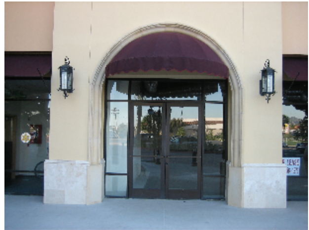
Window and Door Trim
